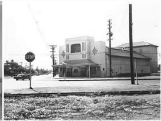
Kahului Theater, just prior to demolition, 1963
